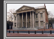
First Bank of the United States Philadelphia, Pennsylvania, USA Bouwjaar: 1791-1797 Architect: Samuel Bladgett
