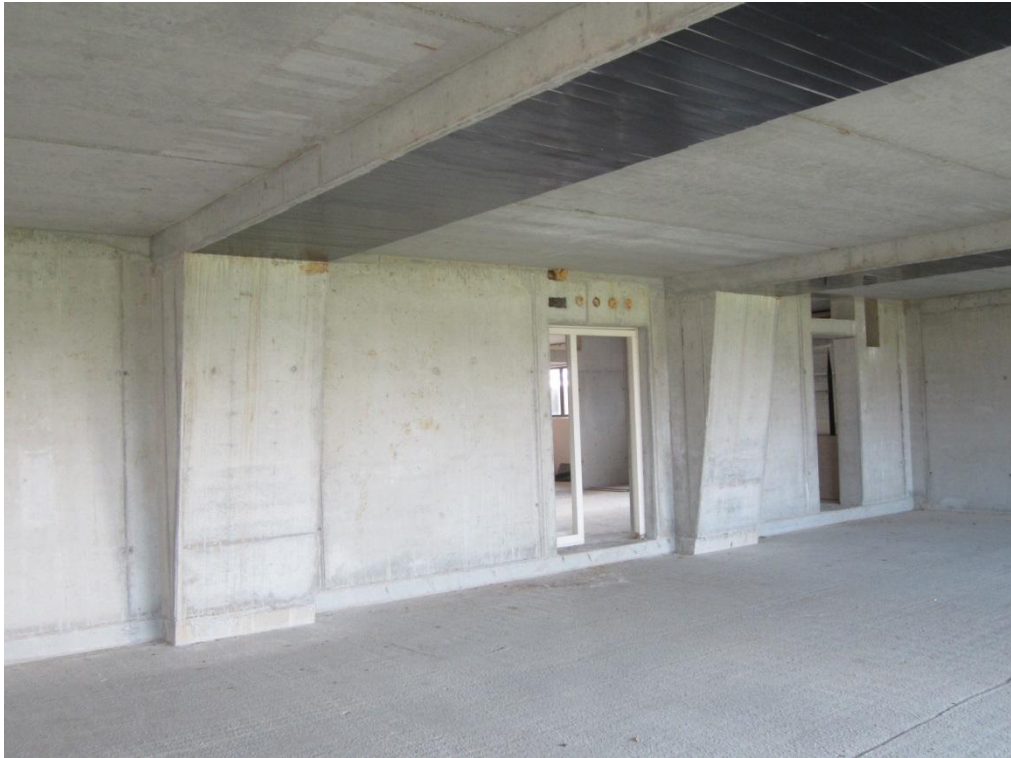
Foto C1: Opening in de stabiliteitswand as 2 en 3
