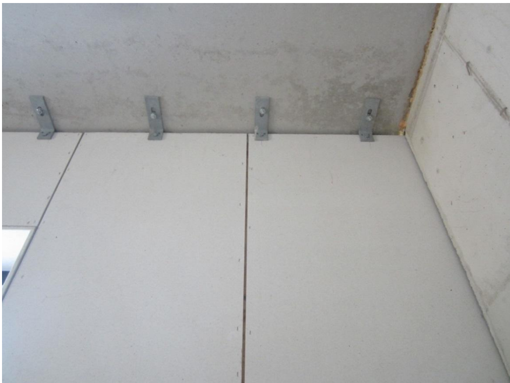
Foto B4: Verankering HSB element
