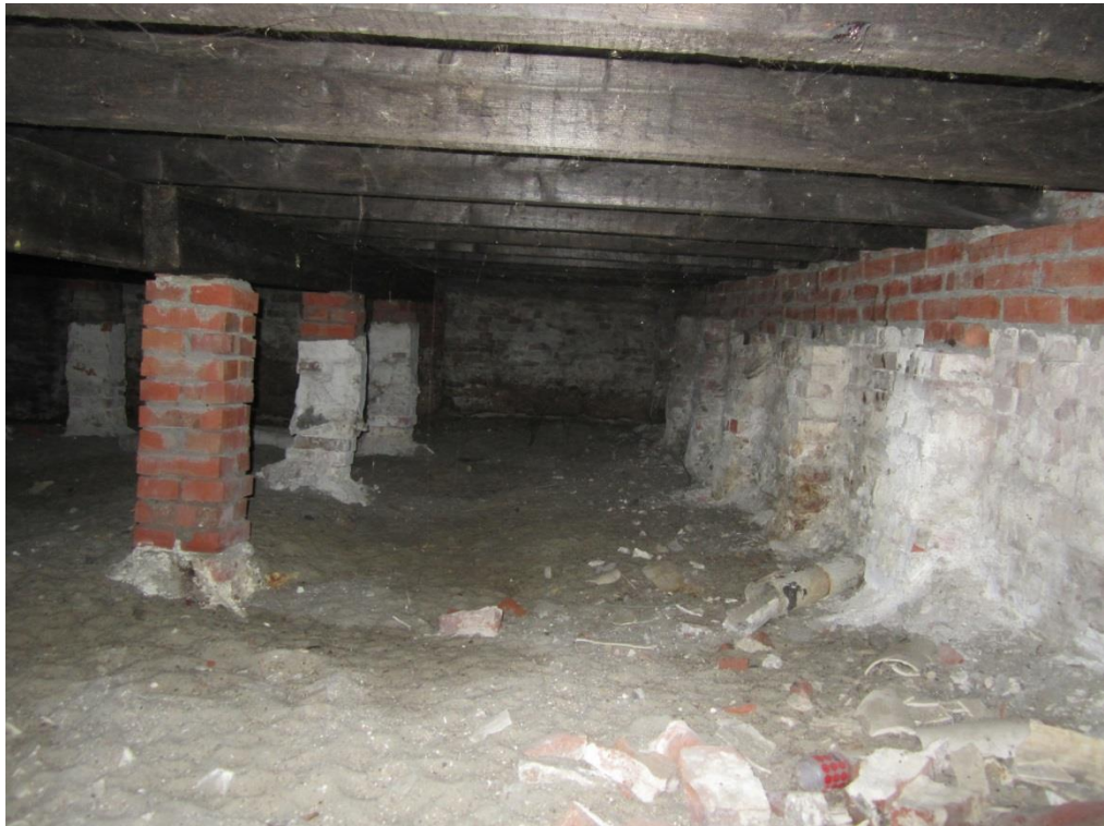
Foto 4: Oplegging houten begane grondvloer
